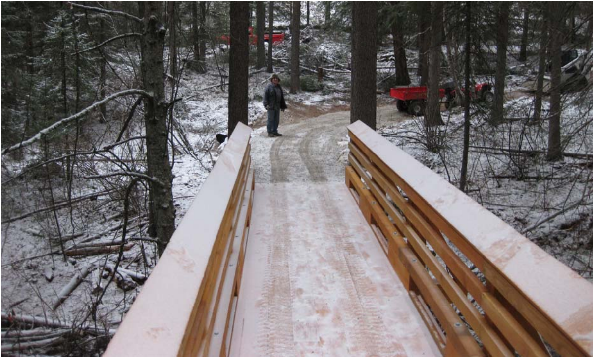
The finished approaches to the bridge
