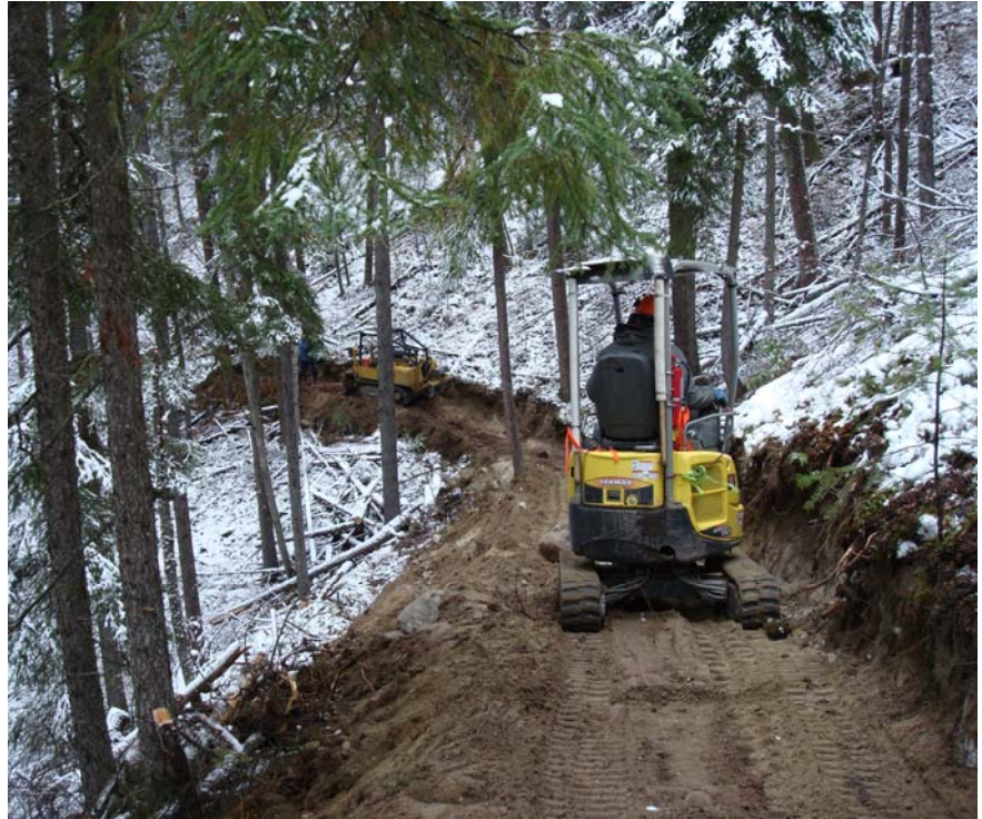
The Sweco dozer and Yanmar mini-excavator work well together
