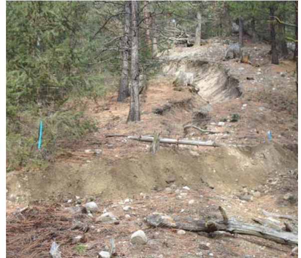
X-ditches channel water into the natural drainages
