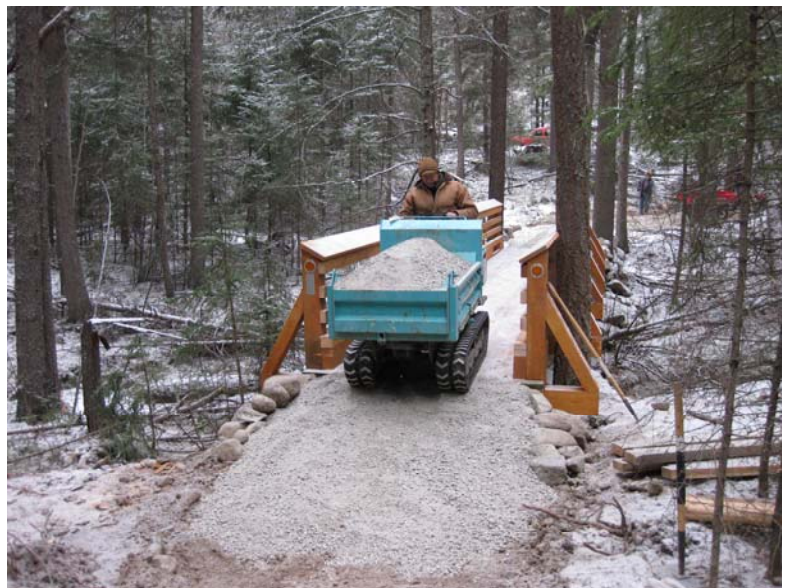
Hauling rock to harden the bridge approaches
