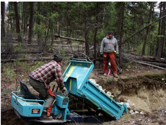
Two of our three crewmembers from Westbank First Nation work on a check dam
