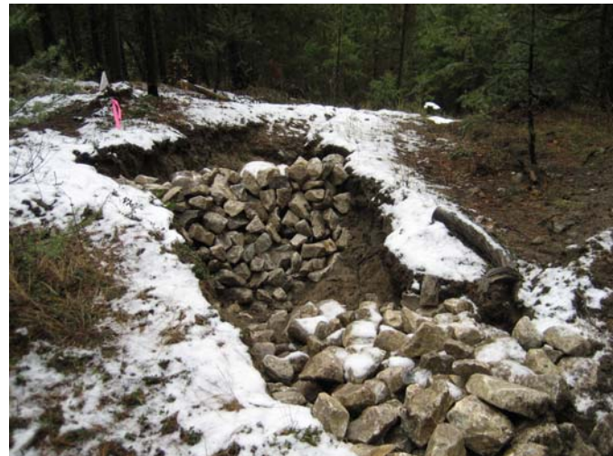
Check dams in an old eroded trail
